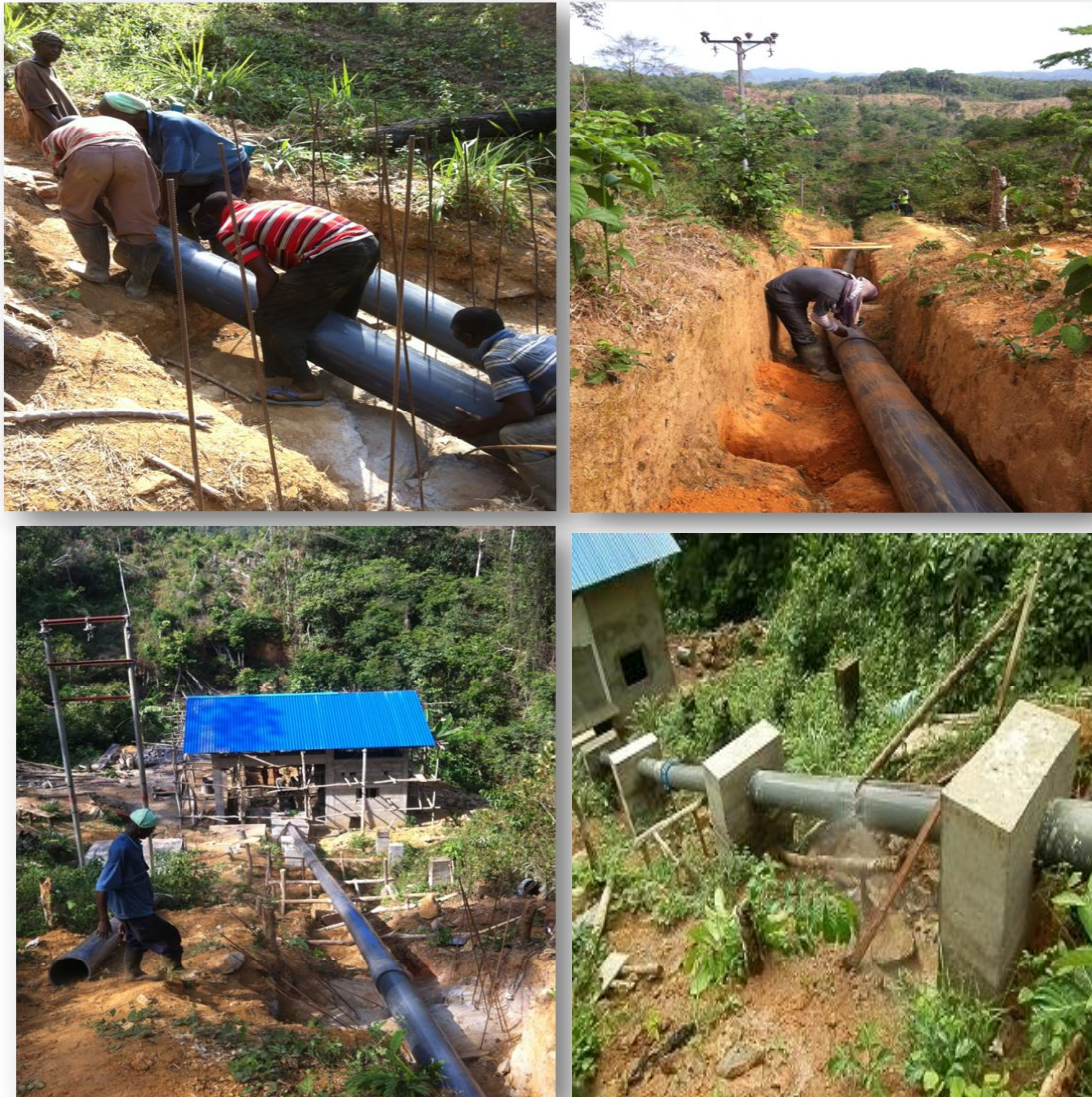
Reconstruction of the Ultra PVC Penstock
