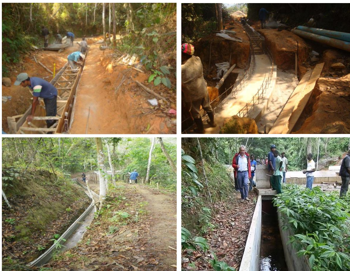
Reconstruction of the Headrace Channel
