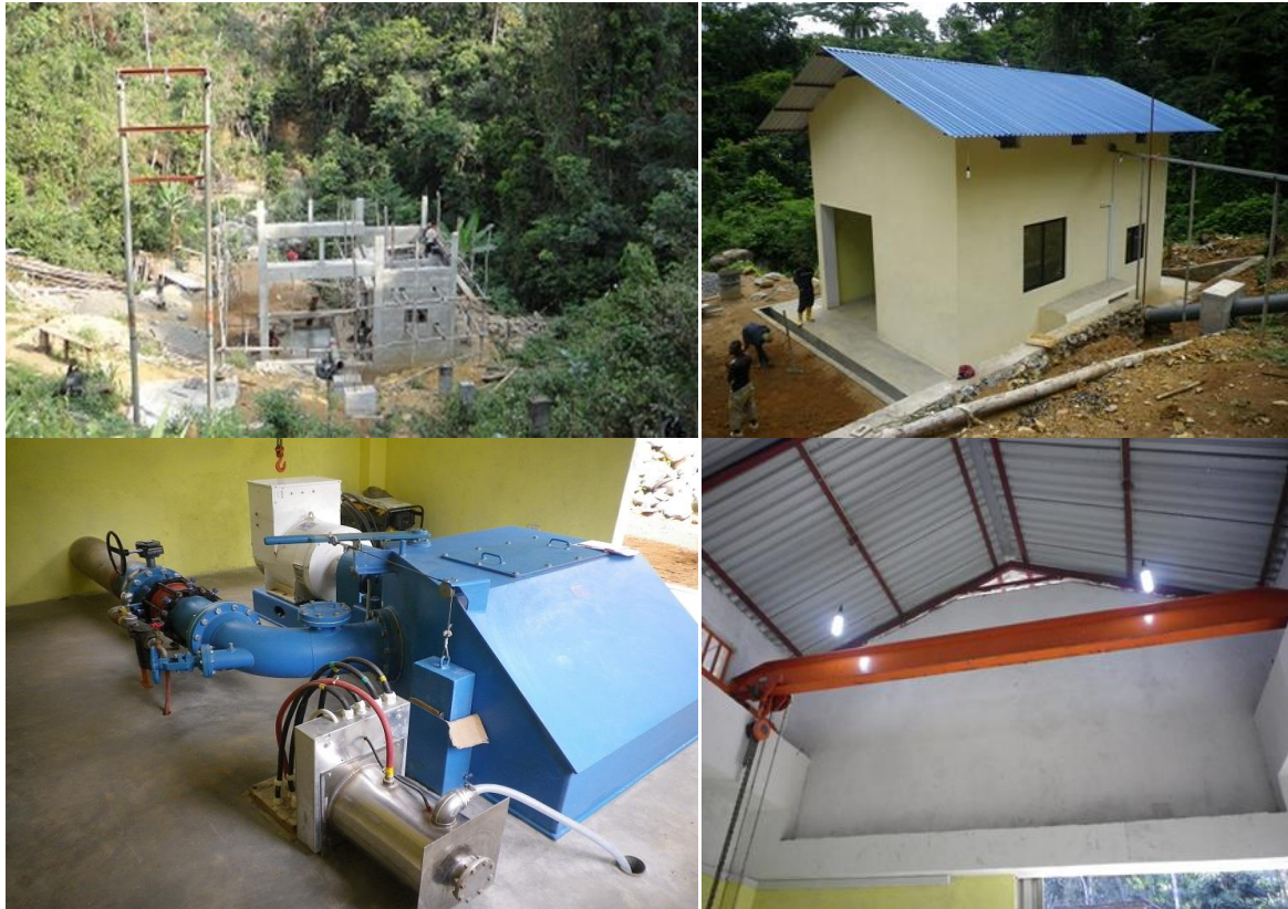
Reconstruction of Single Floor Powerhouse
