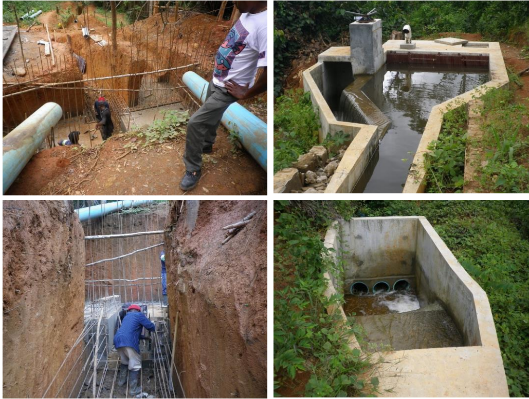
Reconstruction of the Forebay Tank and Spillway
