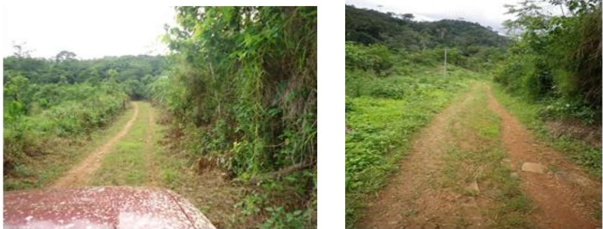
Road from Yandohun Community to hydropower site widened by Community workers
