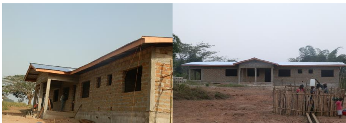
Ongoing Construction of the Guesthouse
