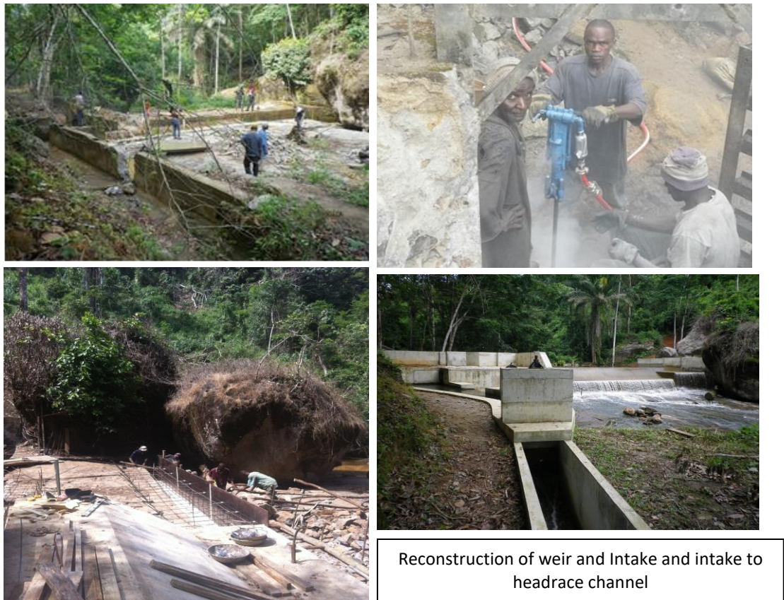
Figure 3: Reconstruction of the weir and intake to headrace channel
